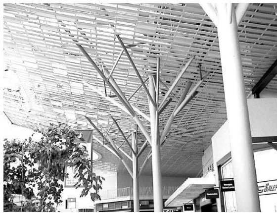
Figure 1 : Centre commercial Auchan, France
